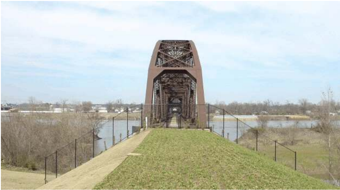
The old Rock Island Sunbelt Route (Choctaw Route) bridge across the Arkansas River March 4, 2005. The Clinton Presidential Center is to my right and behind me. They are going to make this bridge a pedestrian bridge by 2007. The Choctaw Passenger Terminal remains, and is to my left. ( Ken Ziegenbein photo )
