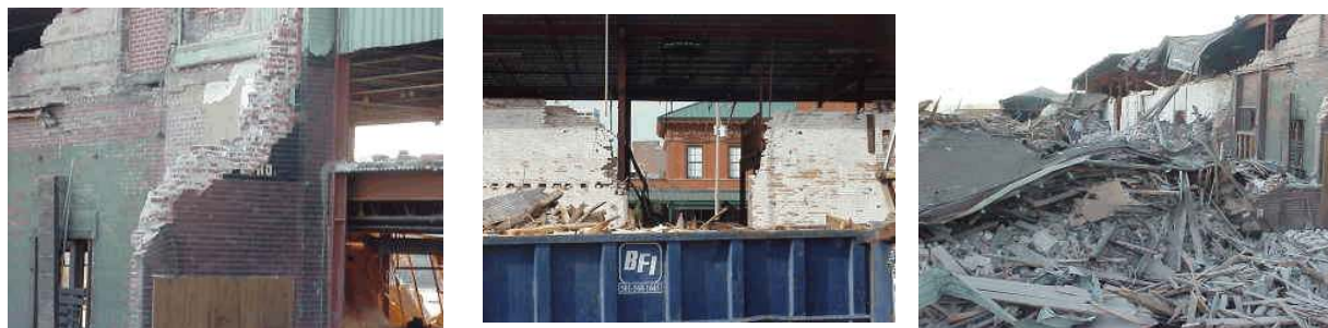
A few photos on the day of the demolition, Nov 21, 2001
