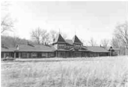
Oklahoma Row cottage, built in 1904 at Monte Ne, on a knoll overlooking Silver Spring. ( Corps of Engineers photo, Clifton E. Hull collection )
